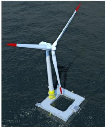
2 MW wind turbine to be fitted on the concrete floating foundation featuring the Damping Pool® system designed by Ideol
