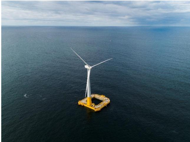
The connection of the electricity export cable and a final series of tests carried out in recent days enabled the Floatgen wind turbine, which is installed 22 km off Le Croisic (Loire-Atlantique), to become fully operational on Tuesday 18 September.
